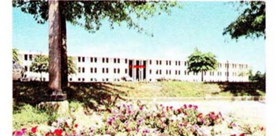
As part of its celebration of twenty-five successful years in America, Canon U.S.A., Inc. has moved its Headquarters to a new prestigious address—One Canon Plaza, Lake Success.
